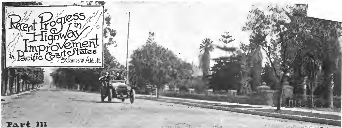
One of the Beautiful Boulevards of the City of Los Angeles, Cal., That Has Been Treated by the Petrolithic Process.
